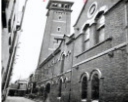
B0128 Old Fire Brigade Tower.jpg
