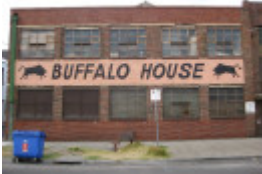
Buffalo House - 3-5 Union Street, Brunswick
