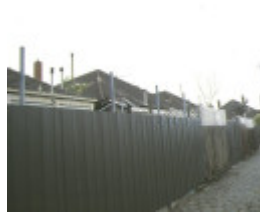
108 116 gladstone street south melbourne rear lane view
