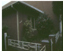
108 116 gladstone street south melbourne iron fence
