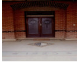
AP 02-1 - detail of doors opening onto verandah - Shire of Northern Grampians - Stage 2 Heritage Study, 2004
