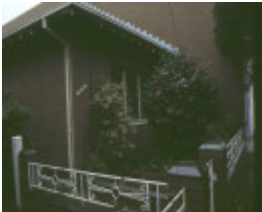
108 116 gladstone street south melbourne iron fence
