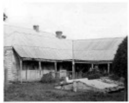
CB 05 3 - Undated photograph, State Library of Victoria Picture Collection - now demolished
