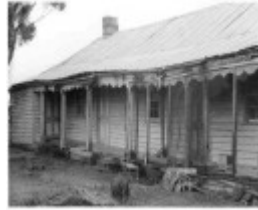
CB 05 2 - Undated photograph, State Library of Victoria Picture Collection - now demolished
