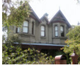
St Martin's Anglican church vicarage
