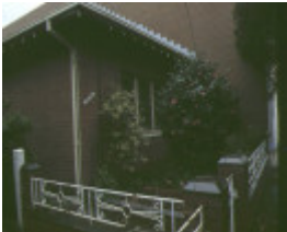
108 116 gladstone street south melbourne iron fence
