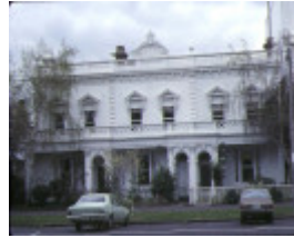
1 terrace 47 howe cres south melb front view
