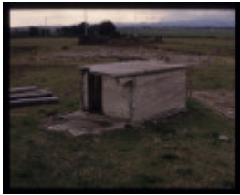
WONTHAGGI NO.18 SHAFT (NO. 4 BENCH, EASTERN AREA)
