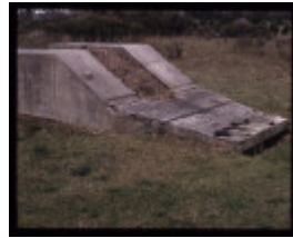
WONTHAGGI NO.18 SHAFT (NO. 4 BENCH, EASTERN AREA)
