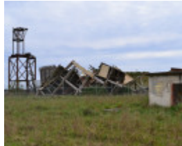
Wonthaggi Kirrak Area- Collapse Sept 2012
