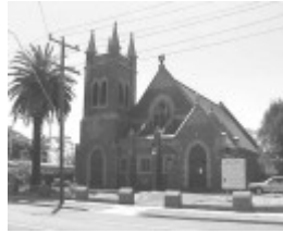
Site 043 - HV McKay Memorial Presbyterian Church.jpg
