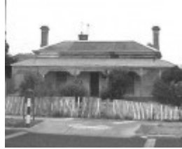
Site 093 - St Albans estate - 16 Arthur Street.jpg
