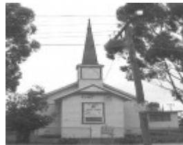
Site 094 - St Albans Uniting Church.jpg
