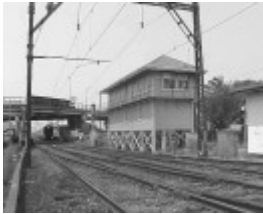
Site 026 - Sunshine railway signal box.jpg
