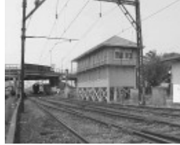
Site 026 - Sunshine railway signal box.jpg
