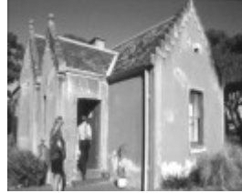
Site 017 - Overnewton gatehouse.jpg
