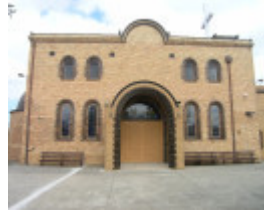
HO119 St Andrews St Greek Orthodox Church.JPG
