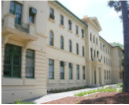
FORMER VICTORIA POLICE DEPOT SOHE 2008
