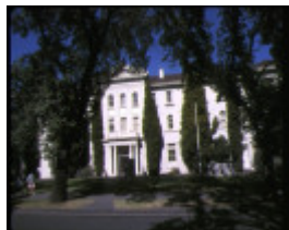
1 former Victorian police mounted branch depot St Kilda Road Southbank front entrance
