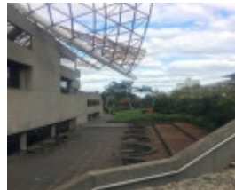
2019_Rear of Theatres Building.jpg
