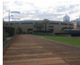
2019_Walkway rear of Forward Surge.jpg
