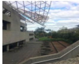
2019_Rear of Theatres Building.jpg
