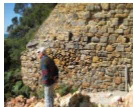
Bell Point Lime Kiln, September 2011
