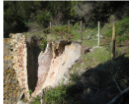
Bell Point Lime Kiln, September 2011
