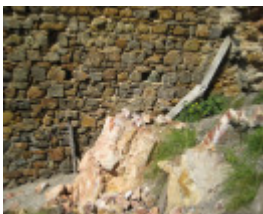
Bell Point Lime Kiln, September 2011
