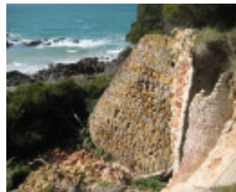
Bell Point Lime Kiln, September 2011
