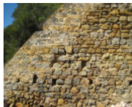
Bell Point Lime Kiln, September 2011
