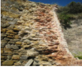
Bell Point Lime Kiln, September 2011
