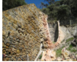
Bell Point Lime Kiln, September 2011
