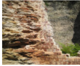
Bell Point Lime Kiln, September 2011
