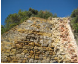
Bell Point Lime Kiln, September 2011
