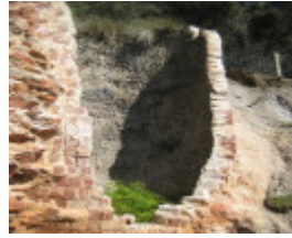
Bell Point Lime Kiln, September 2011
