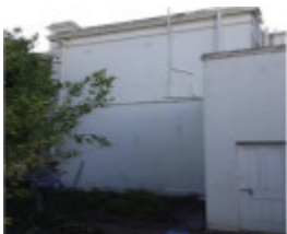
Before Photograph - Reference F3856 2014
