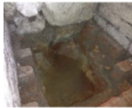
Before Photograph - Reference F3856 2014
