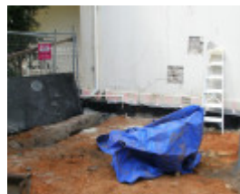
During Photograph - Reference F3856 2015
