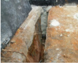
During Photograph - Reference F3856 2015
