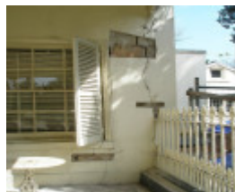
During Photograph - Reference F3856 2015
