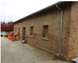
During Photograph - Reference F3879 2015
