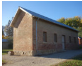
Before Photograph - Reference F3879 2014
