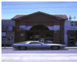
1 former south yarra railway station toorak road south yarra front view
