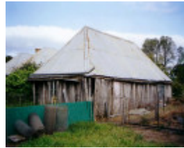
MAW 01 1 - Photograph, vertical timber slab building at the rear of the homestead represents one of the earlier parts of the complex - Shire of Northern Grampians - Stage 2 Heritage Study, 2004
