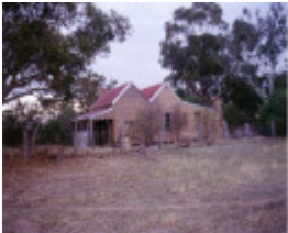
SC 05 - Side view of farm house - Shire of Northern Grampians - Stage 2 Heritage Study, 2004
