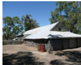
TOTTINGTON HOMESTEAD, STONE COTTAGE AND WOOLSHED SOHE 2008
