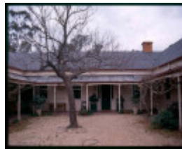
H0305 Tottington Homestead courtyard
