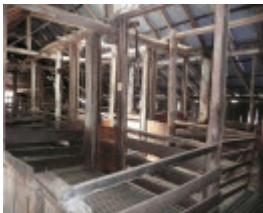
TOTTINGTON HOMESTEAD, STONE COTTAGE AND WOOLSHED SOHE 2008
