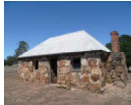
TOTTINGTON HOMESTEAD, STONE COTTAGE AND WOOLSHED SOHE 2008
