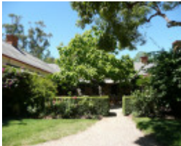
TOTTINGTON HOMESTEAD, STONE COTTAGE AND WOOLSHED SOHE 2008
