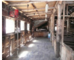
TOTTINGTON HOMESTEAD, STONE COTTAGE AND WOOLSHED SOHE 2008
