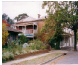
SD 080c - Photograph, side view showing verandah.
