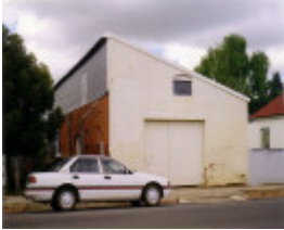
SD 098 - Former Coffee Palace stables, McMahon Street, ST ARNAUD
