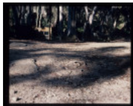
ECHO POINT FOOTINGS
