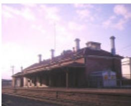
1 st arnaud railway station avenue st arnaud trackside view may1995
