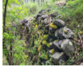
Retaining wall near sluced ground
