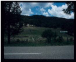
BARWIDGEE CREEK MECHANICS INSTITUTE
