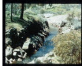
OSBORNE'S FLAT DIVERSION SLUICE
