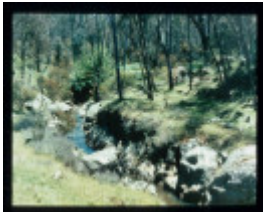
OSBORNE'S FLAT DIVERSION SLUICE
