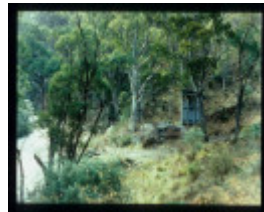
VICTORIA FALLS HYDRO-ELECTRIC POWER STATION
