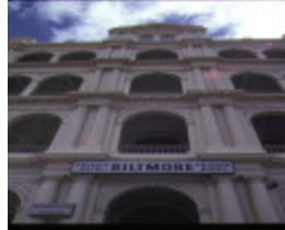
biltmore bridport street albert park front elevation nov1979
