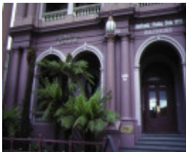
biltmore bridport street albert park front entrance
