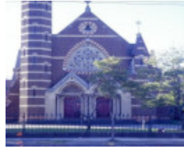
h00864 1 st georges uniting church chapel street st kilda front view she project 2003
