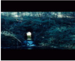
HOUGHTON'S/MCCOY'S FLAT DIVERSION TUNNEL
