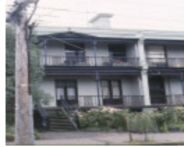
1 eden terrace dalgety street st kilda front view
