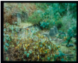
MT MURPHY WOLFRAM TREATMENT WORKS - LOWER WORKS
