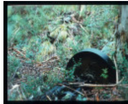
MT MURPHY WOLFRAM TREATMENT WORKS - LOWER WORKS
