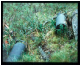
MT MURPHY WOLFRAM TREATMENT WORKS - LOWER WORKS
