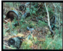
MT MURPHY WOLFRAM TREATMENT WORKS - LOWER WORKS
