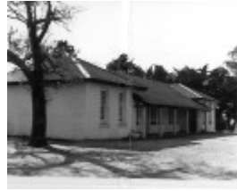
Administration Building, Lake Tyres Aboriginal Mission
