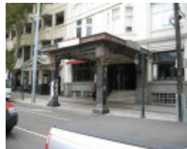
H0706 George Hotel St Kilda 1925 Fitzroy Street entrance to hotel 2009
