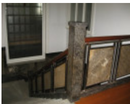
H0706 George Hotel St Kilda 1925 wing stair detail at first floor 2009
