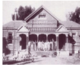
SD 127 1 - During construction. Photograph taken from St. Arnaud, A Pictorial Journey - Shire of Northern Grampians - Stage 2 Heritage Study, 2004
