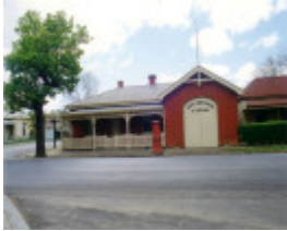
SD 130a - St. Arnaud Fire Station & Turncocks residence
