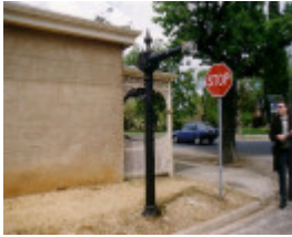
SD 133a - Stand Pipe, Napier Street, corner Inkerman Street, ST ARNAUD
