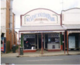
SD 148 - Shop, 'St. Vincent De Paul' (Former ABC Grocery), 35 Napier Street, ST ARNAUD
