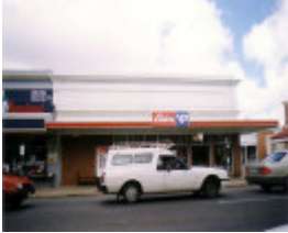
SD 151 - Former McBride building, 51 Napier Street, corner Raglan Street, ST ARNAUD
