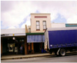
SD 160a - Two-storey building (former Mewkells Chemist shop), 71 Napier Street, ST ARNAUD
