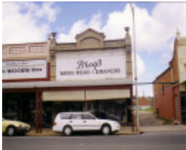
SD 180a - Shop - Brays Store, 115 Napier Street, ST ARNAUD
