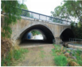
KINGS BRIDGE, OVER BENDIGO CREEK SOHE 2008
