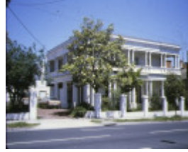
1 berkeley hall princess street st kilda front view
