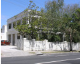
BERKELEY HALL SOHE 2008
